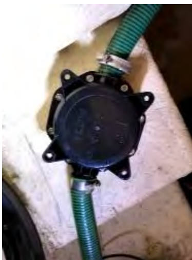
Fig 3 – New pump installed as seen inside cabin
