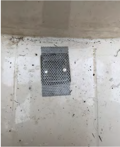
Figs 5 & 6 – Cockpit sump strum box
