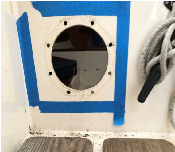
Fig 1 – pump mounting holes enlarged to suit new pump
